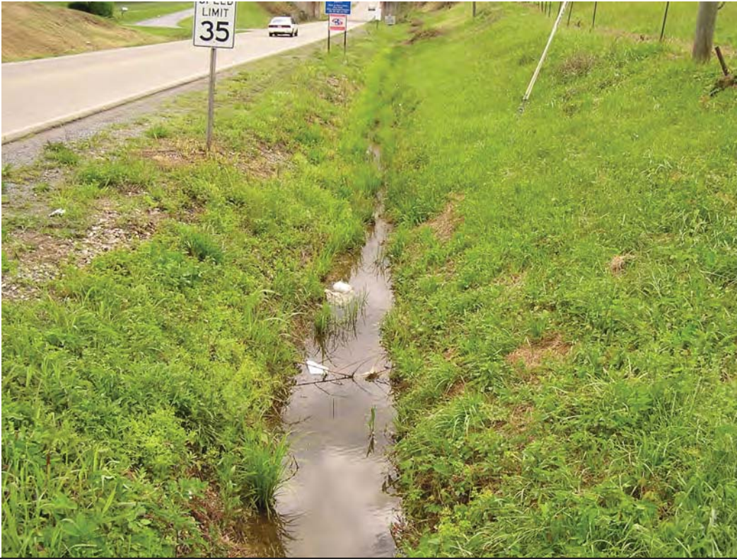
Photo 3: STA 103+00RT, View of WWC-2 facing east.
