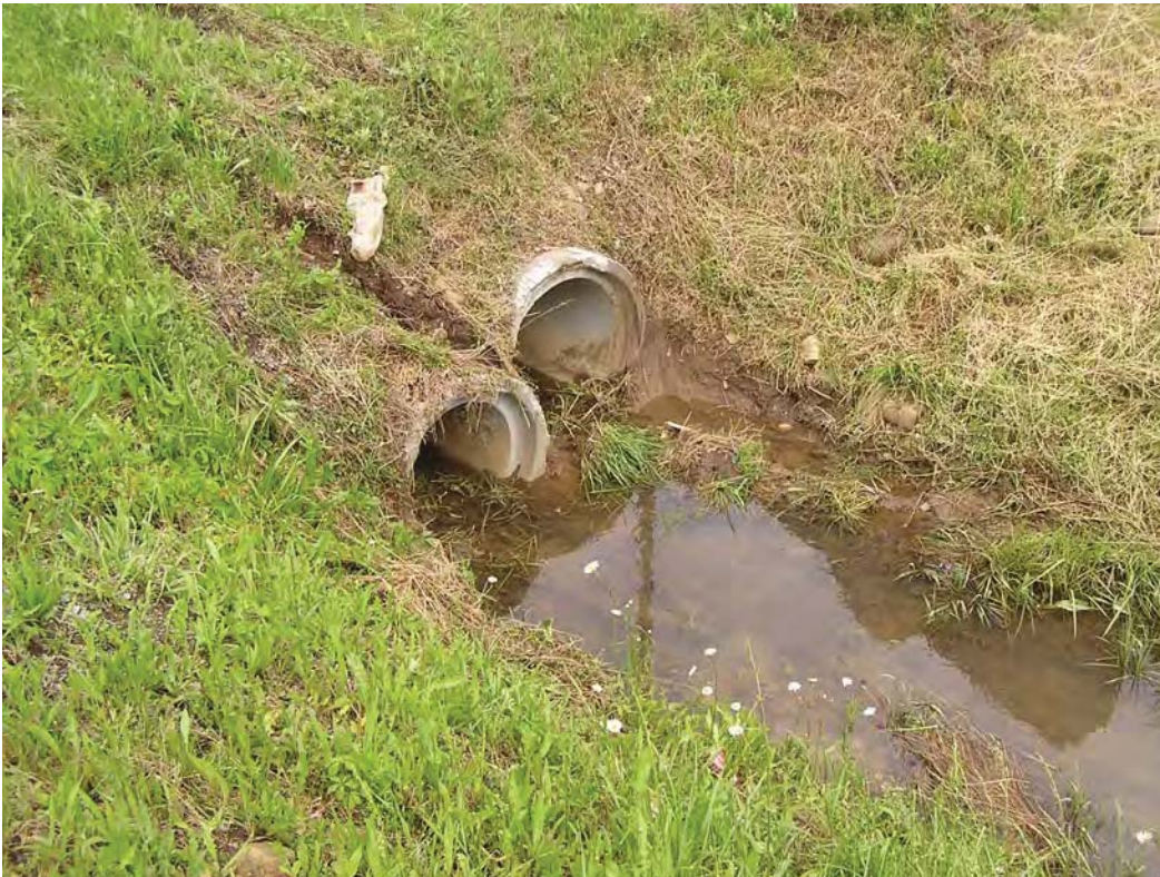
Photo 4: STA 101+00 LT, View of WWC-3 facing north.
