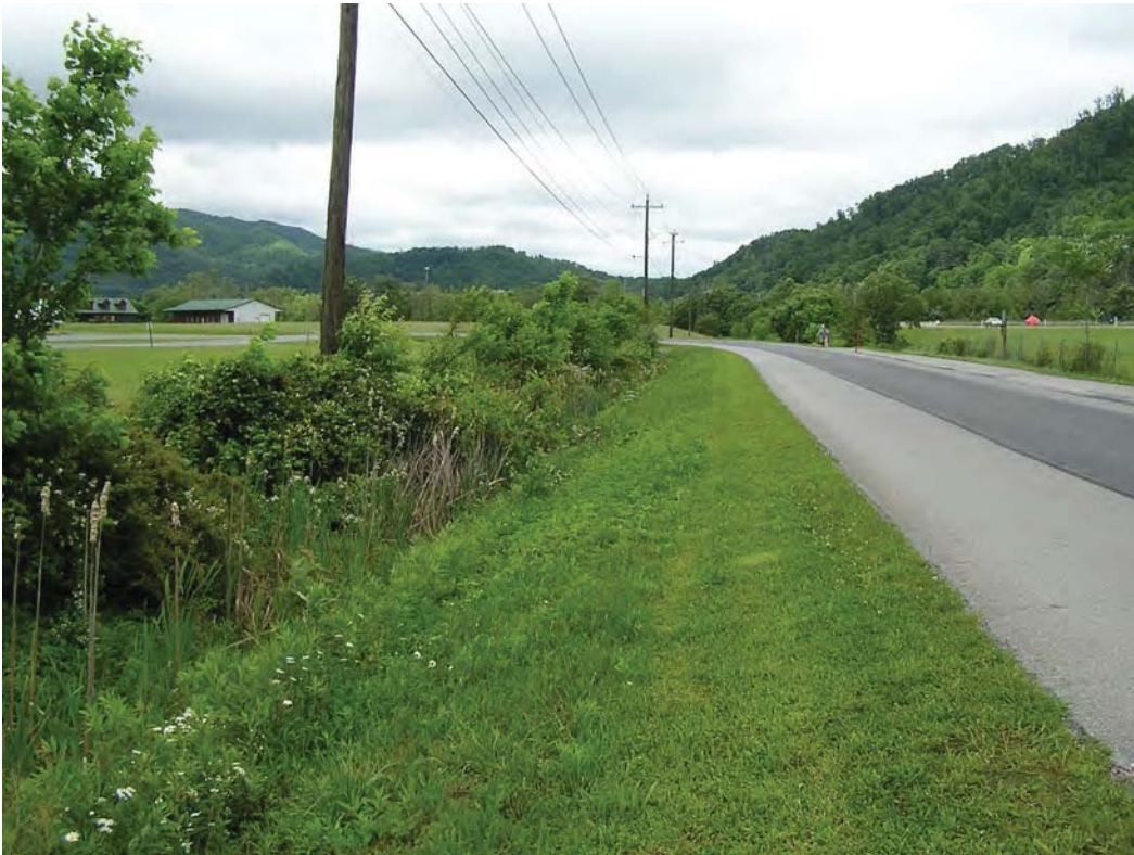
Photo 6: STA 25+00 RT View of WTL-1 facing northeast.
