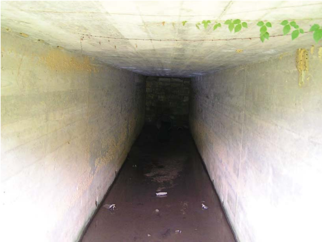
Photo 2. STA 101+25LT, View of WWC-1 facing south.
