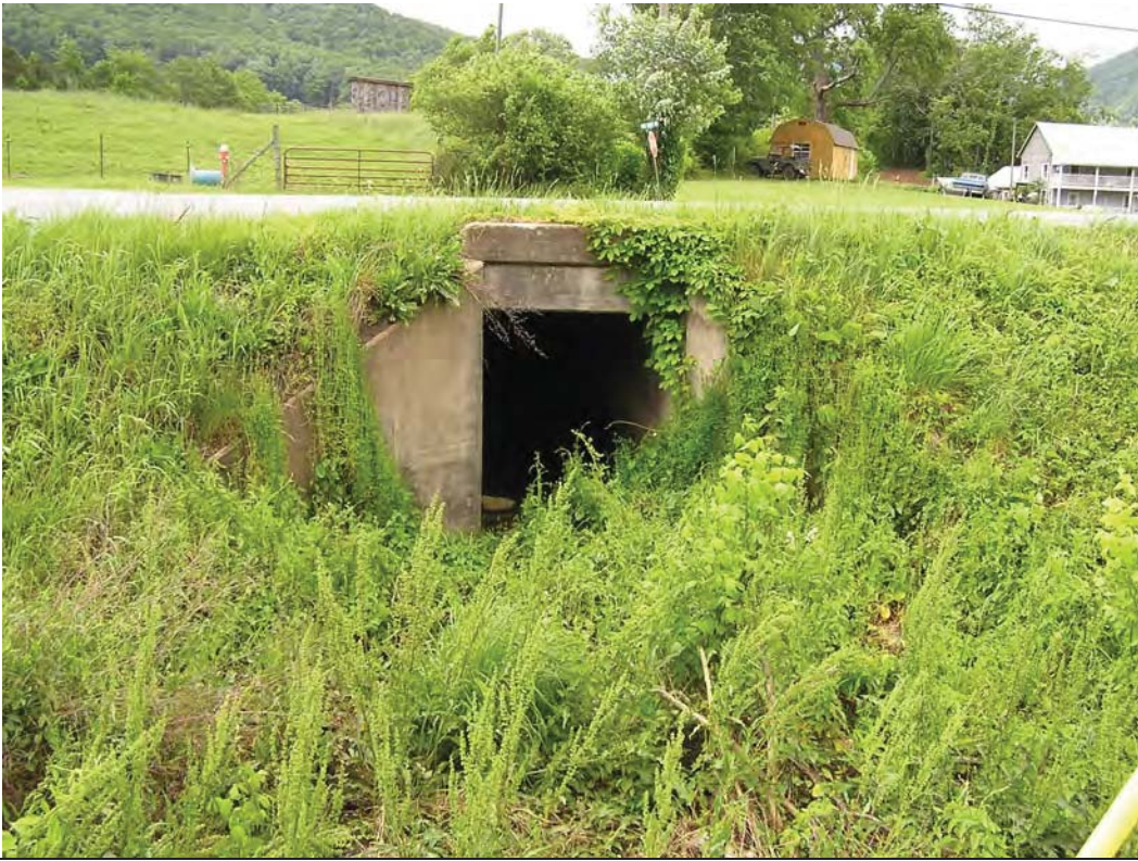
Photo 1: STA 101+25LT, View of WWC-1 facing south.
